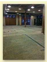
The slab in the 103-year-old building bore evidence of many past lives. It was of different colors, had cracks and heaves, and was covered in layers of mastic.
