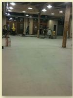
The slab is smooth after grinding and is ready for densification and polishing. The crew used a colloidal slica-based densifier to speed up the process and to optimize the surface.
