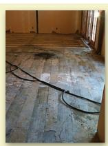
During the first grinding pass, the slab is ground in interlaced stripes to keep the depth even. Evidence of its deteriorated condition is plentiful.
